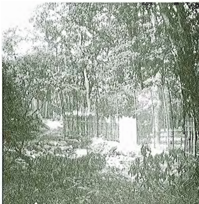
The mesh is fixed to the bent pipes. These poles were especially developed by the architect blending with the trees by their slim upright form and conserving tree roots by their special anchoring
