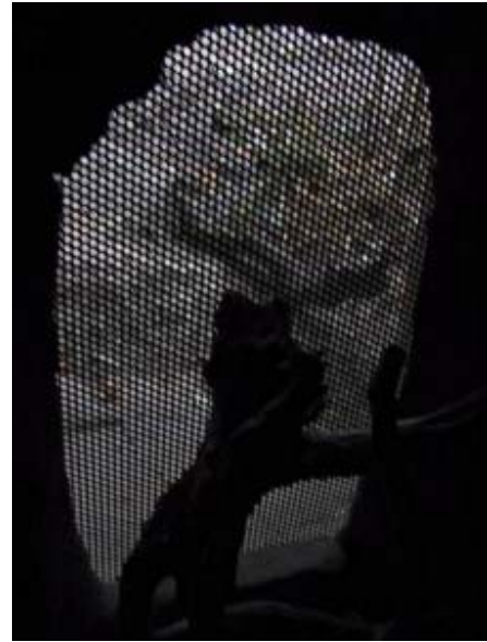
Perforated Screen - The perforated metal panel makes it possible for the visitors to see, hear and smell the tigers close up. The holes are so small that no tiger claw or child finger fits through. ©Monika Fiby, 2004
