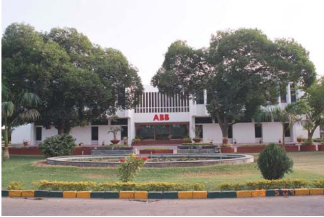
Image 1. Main Office Building of Asian Brown Boveri
